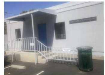
Maintenance and Operations Located at 2121 16th Street West of Corsair Field
